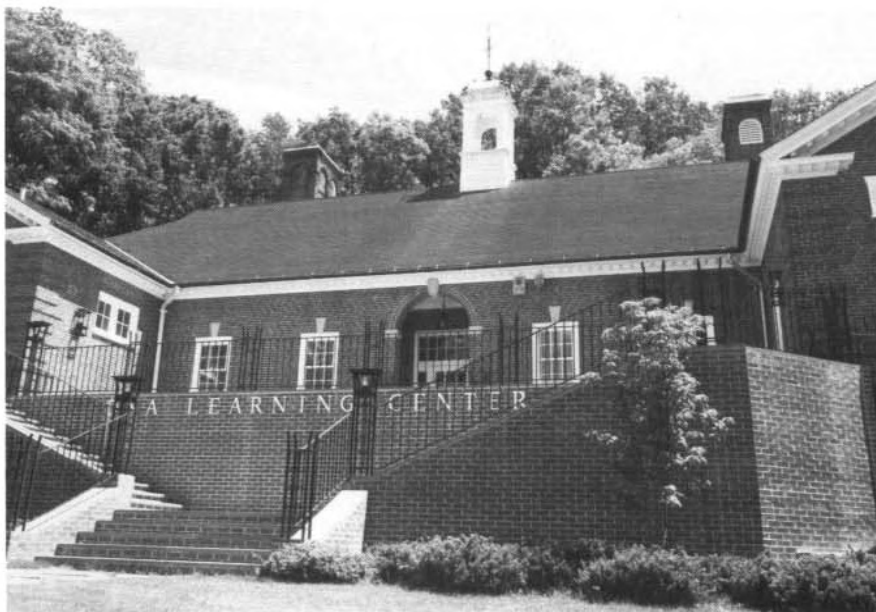
Demolition and reconstruction of front porch of DNALC.
